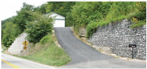
Shales in the Pikeville Formation provide a poor foundation and are unstable on slopes. Hillside construction of roads and homes on shale in Johnson County often requires additional support and drainage management to ensure slope stability. In Whitley County, rock gabions and a chain link fence provide stability to a cut slope in the Pikeville Formation along Doc Siler Road. Photos by Bethany Overfield and Dan Carey, Kentucky Geological Survey.
